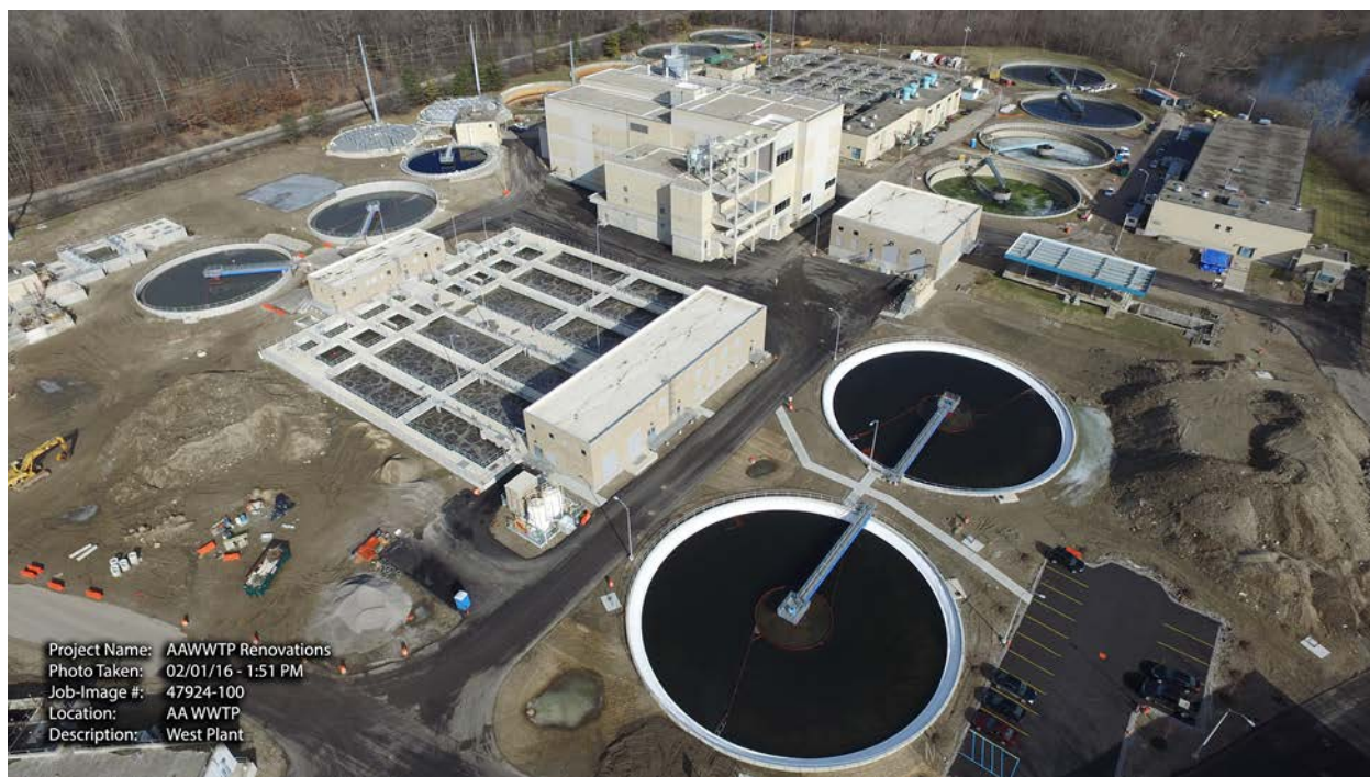
Wastewater Treatment Plant Facilities Renovations Project
